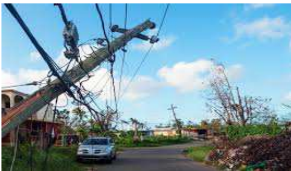
Figure 1: Damage site during the 2017 Hurricane Maria Event in Puerto Rico
