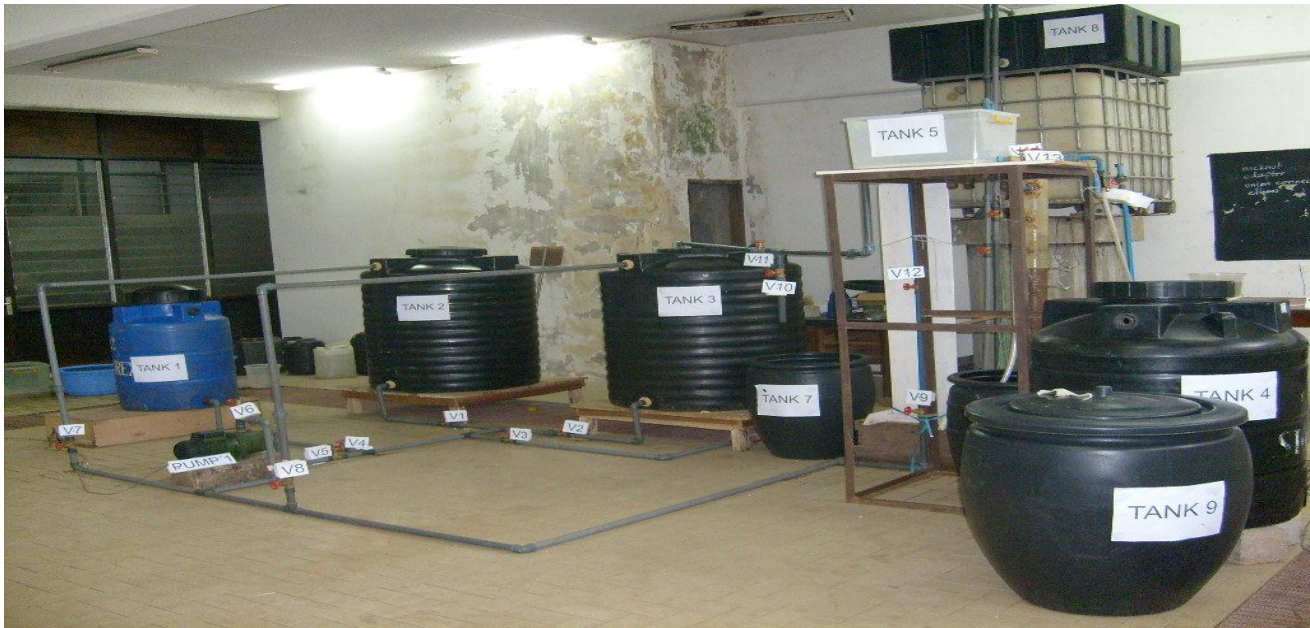
Plate 1: Pipe network for circulating water during the study
